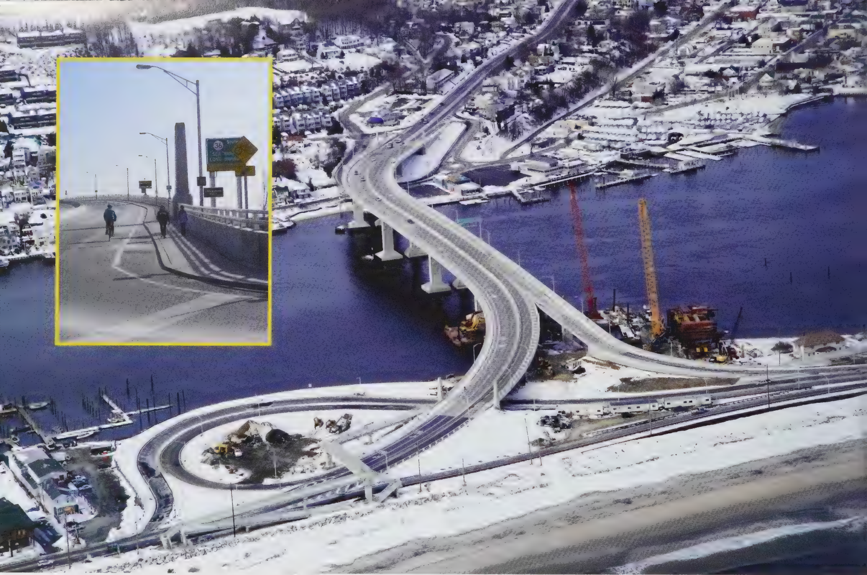
Route 36 Highlands Bridge Replacement (2010)
